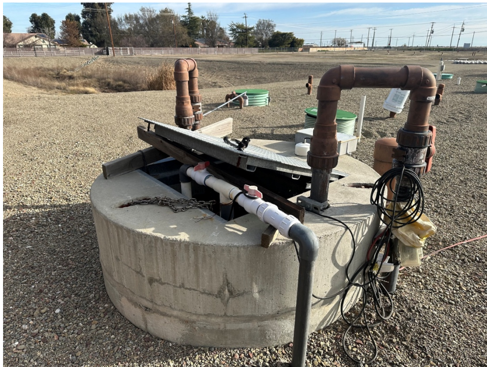
Taken February 21, 2025, underground tank
