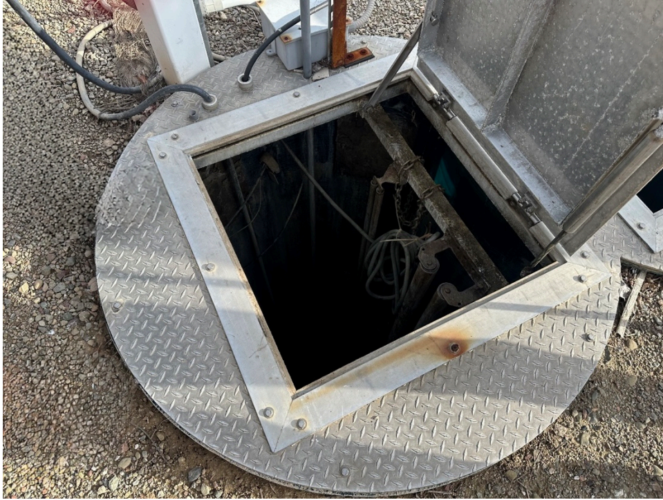
Taken February 21, 2025, underground tank access
