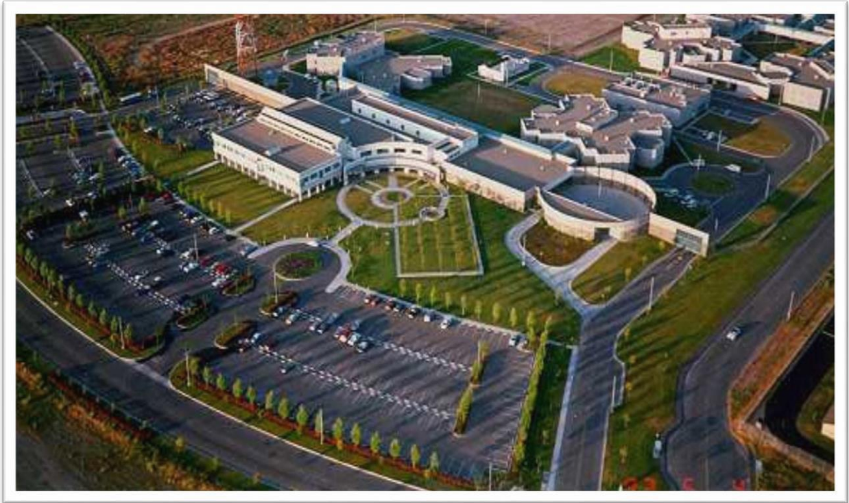
San Joaquin County Jail Complex
